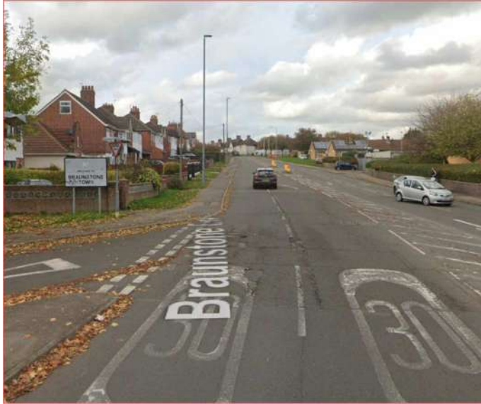
Braunstone Lane after Narborough Road South junction – New Sign
