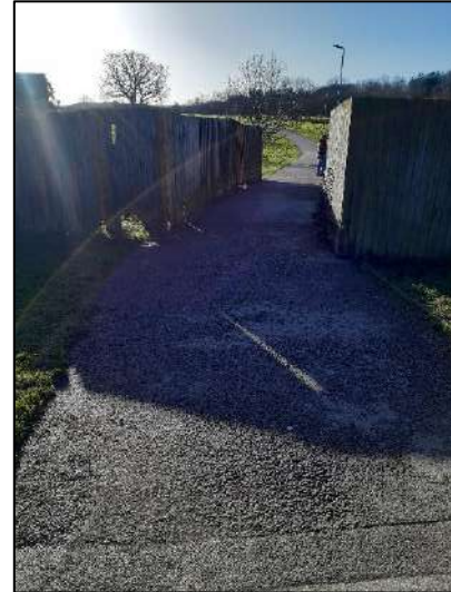
Southbound approach to bridge
