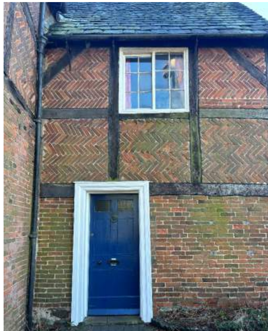
Image 15: The Manor, detail showing herringbone brick pattern, later inserted door and surround and vertical sliding sash window.
