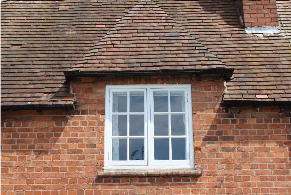
Despite varying elevation treatments, the dwellings at 1-6 Main Street are constructed from red brick, with pitched clay tile roofs and timber casement.
