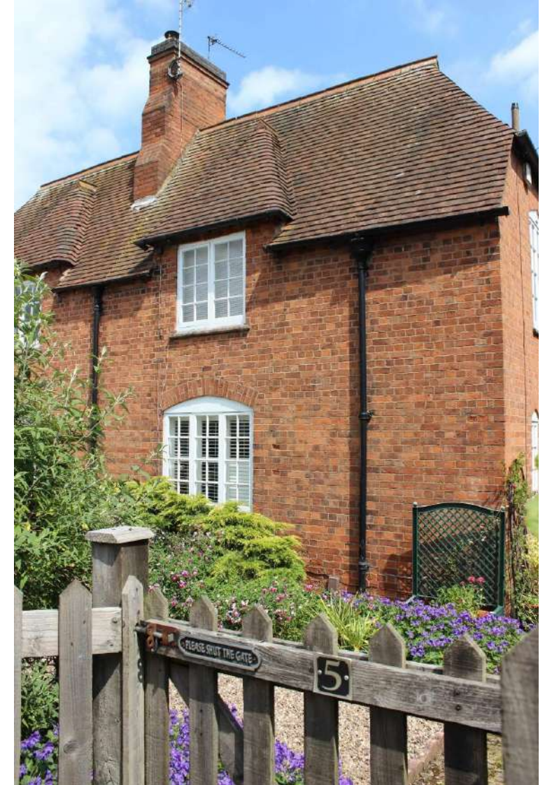
The pair of cottages at 5-6 Main Street is the most architecturally plain of all, but nonetheless of much visual interest and architectural merit.
