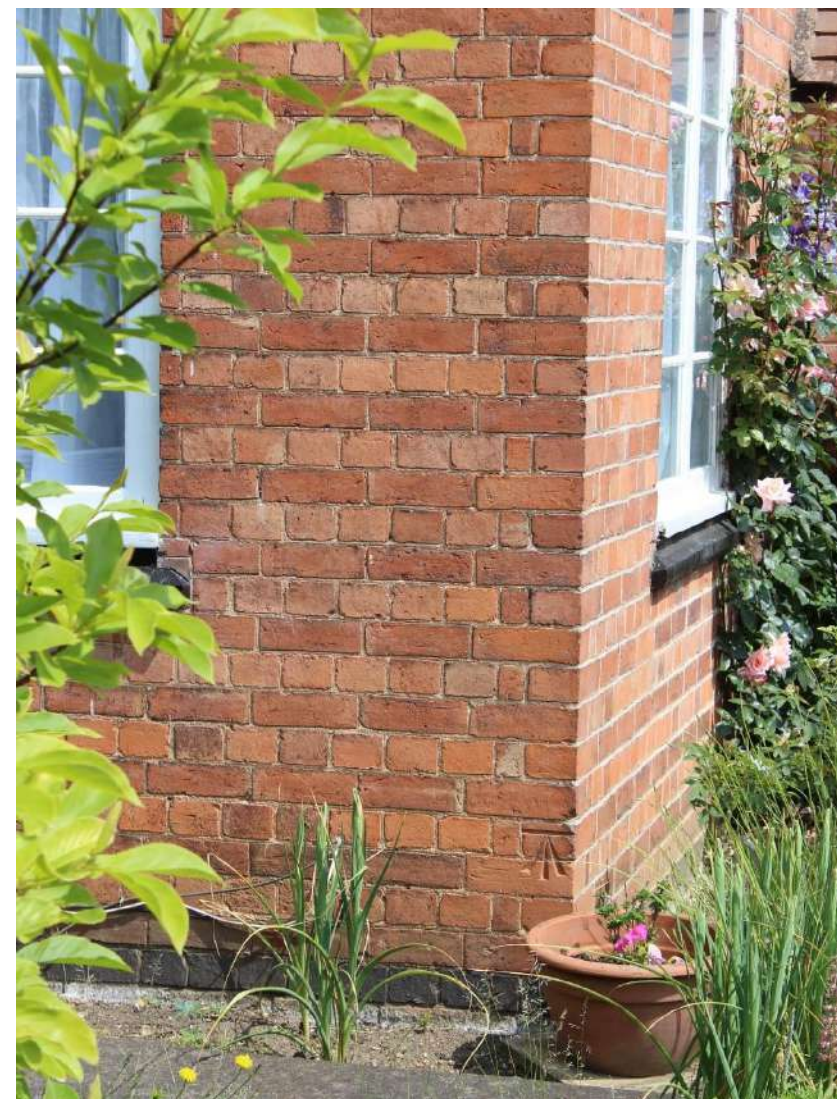
Top: The red brickwork set in Flemish bond with the original stonemason's mark at 3 Main Street.
